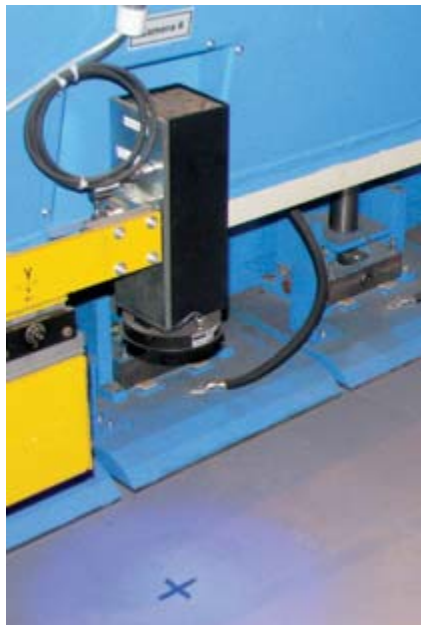
Recognition of markings at the welding station
